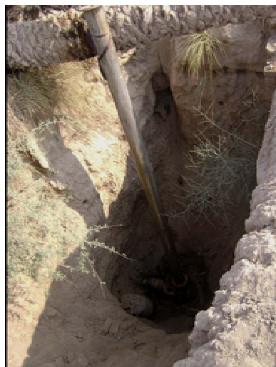
Figure 21: A Bore Pipe for the with drawl of Ground Water in RYK - IE
