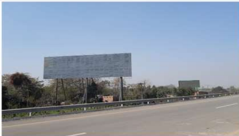
Location: After Ravi Interchange Lahore-Islamabad Motorway
