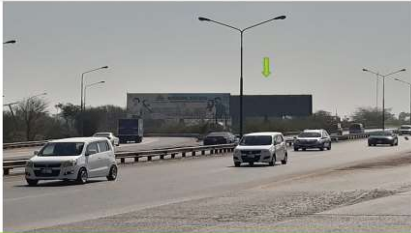
Location: Towards Motorway to Thokar Niaz Baig Multan Road
